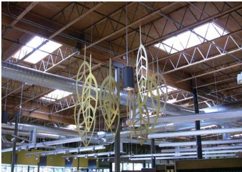
Natural light penetrates skylights and specially glazed street-level windows. The structural ceiling deck in the sales area is the finished ceiling, eliminating other finish ceiling materials.
