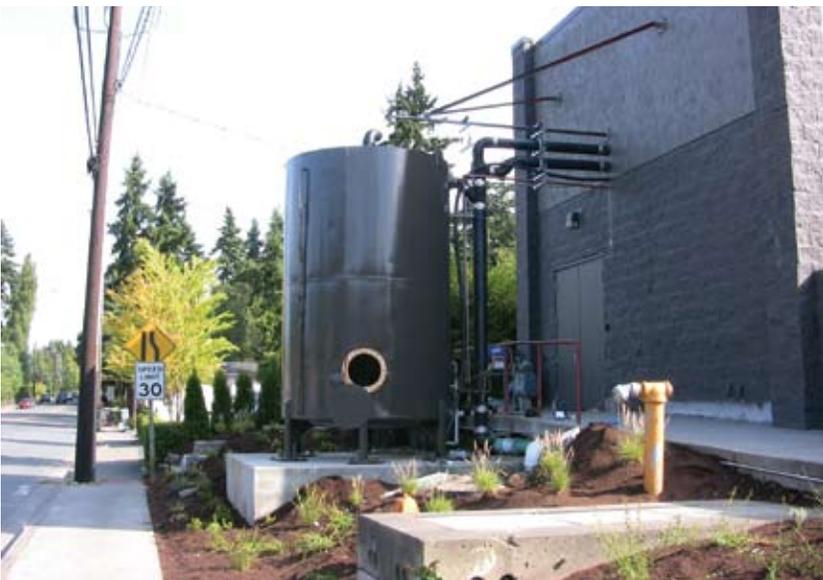
A rainwater harvesting system includes the roof, a 4,500 gallon tank, and a simple system of pipes and filters. Rain gardens capture and clean parking lot water runoff.
